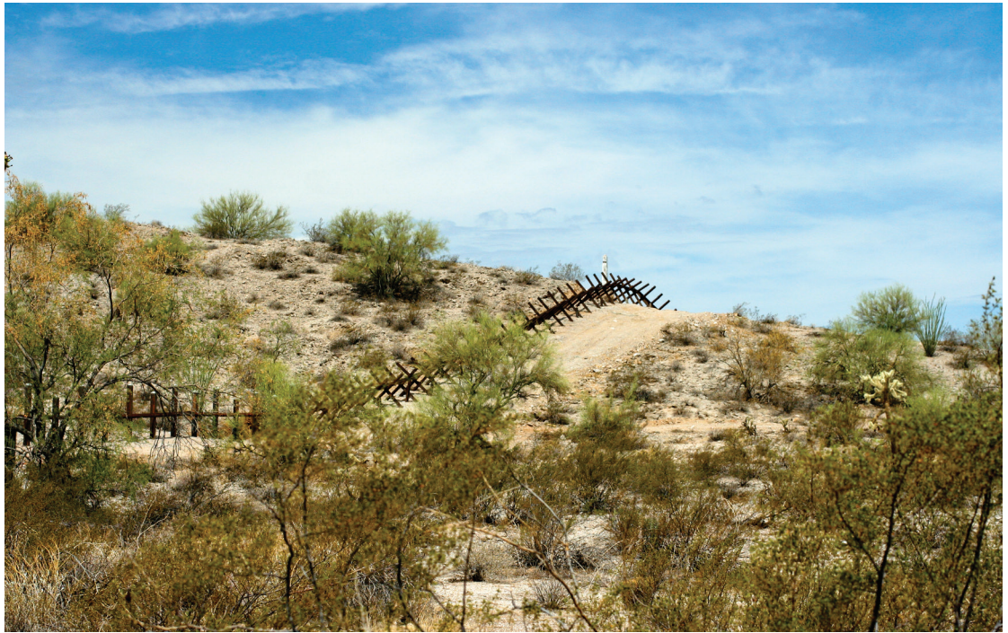
Normandy barrier on US-Mexico border in Organ Pipe National Monument. Chris Clarke photo.
