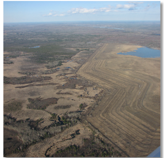
PolyMet's Leaking Tailings Basin
