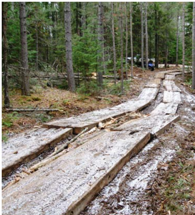
Figure 21. Planking utilized during spring thaw to prevent rutting and compaction
